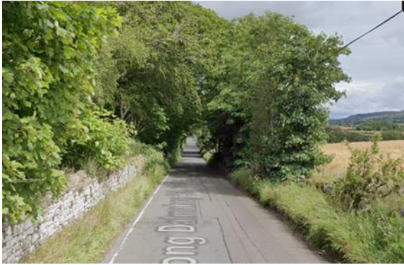
Long Dalmahoy Road Often under 4m wide. Passing safely requires considerable slowing. Frequent accesses in places. Part of National Cycle Network
